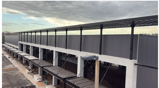
Canopy steel running the tenant storefront line, mid-construction
