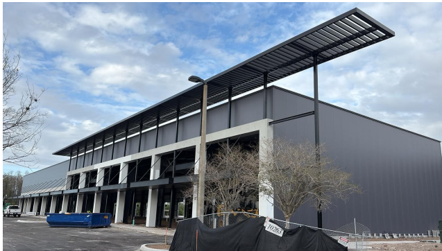
Cantilevered steel storefront canopy and glazed entry
