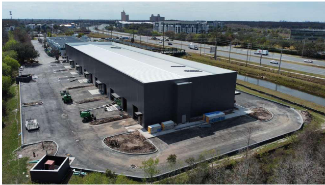
Completed structure, aerial – John Young Parkway frontage
