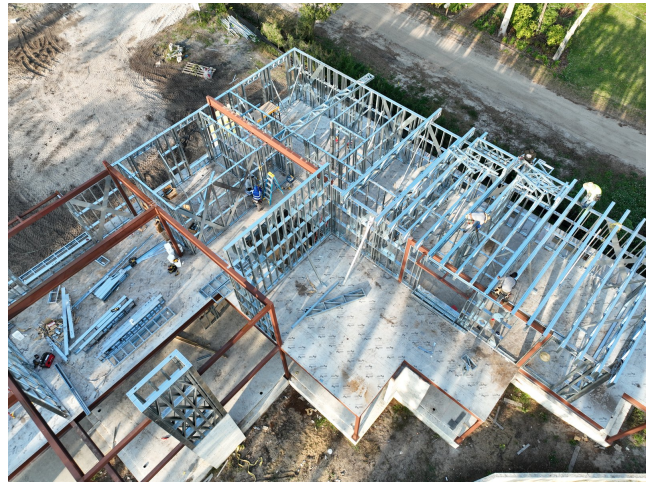
Heavy steel beams carrying light-gauge walls and floor deck
