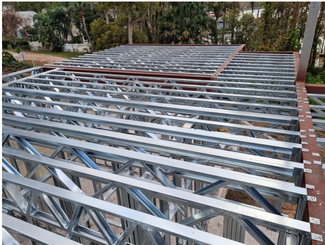
AT Steel LGS open-web floor trusses on a heavy steel support beam
