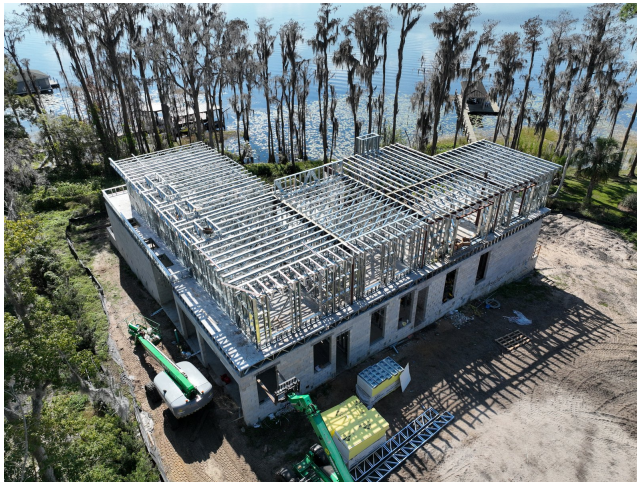
Full LGS floor-truss platform forming the second-floor deck
