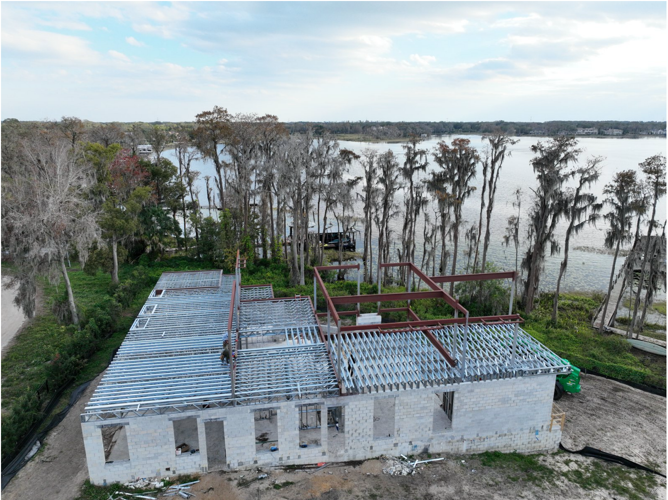
AT Steel framing package erected on site – lakefront residence, Windermere, FL
