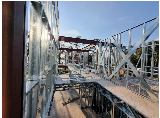
LGS structural walls and heavy steel framing the lake view
