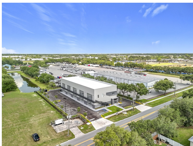
Completed two-level structure, aerial
