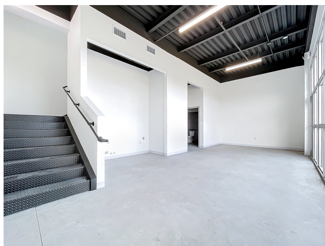
Bracing and mezzanine framing, mid-construction
