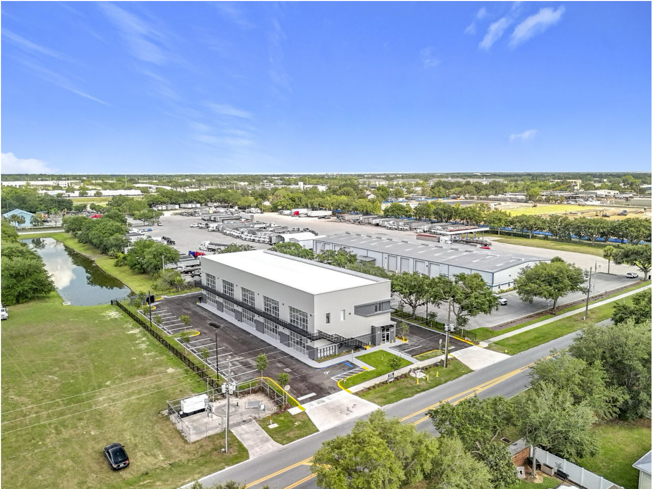
Completed building — 705 Hennis Road, Winter Garden, FL
