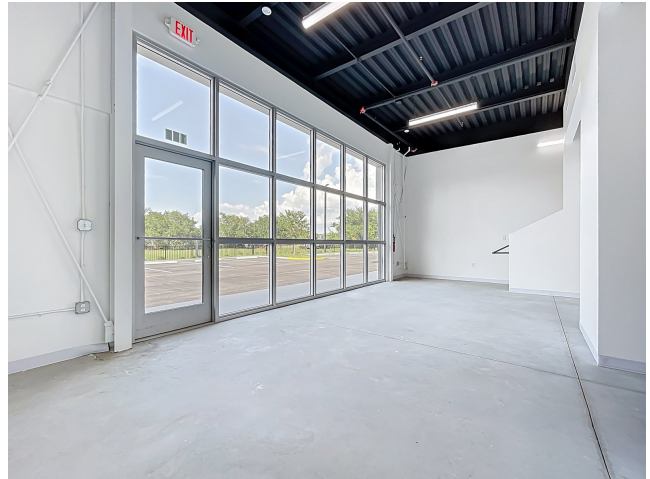
Envelope panels going up
