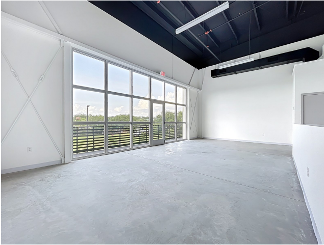
Exposed structural steel, X-rod bracing, storefront glazing
